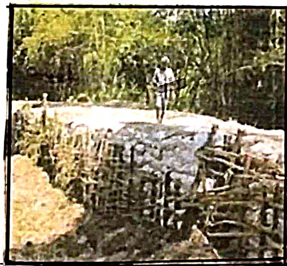
Earthen Embankment with Bamboo fence and sand fill bag.
