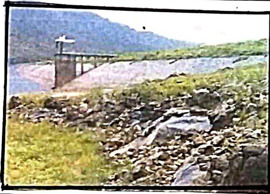
Boulder Pitching embankment.
